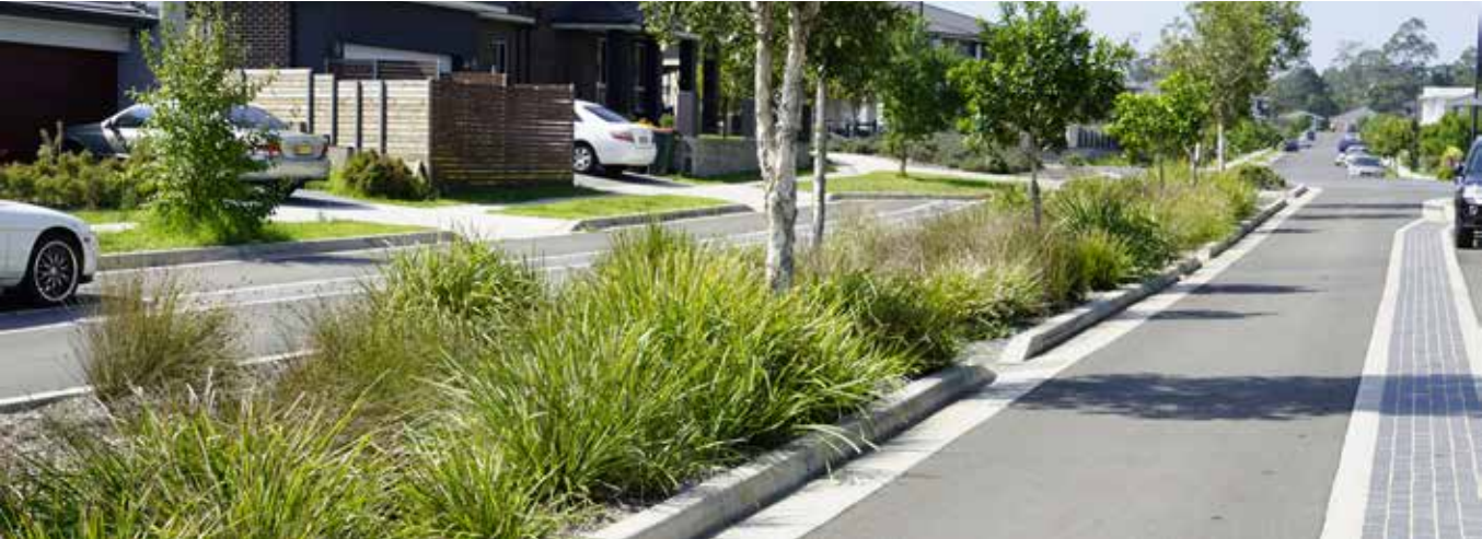
A vegetated swale in a central median strip in Bungarribee, including breaks in the kerb for passive irrigation (Image Credit Blacktown City Council)
