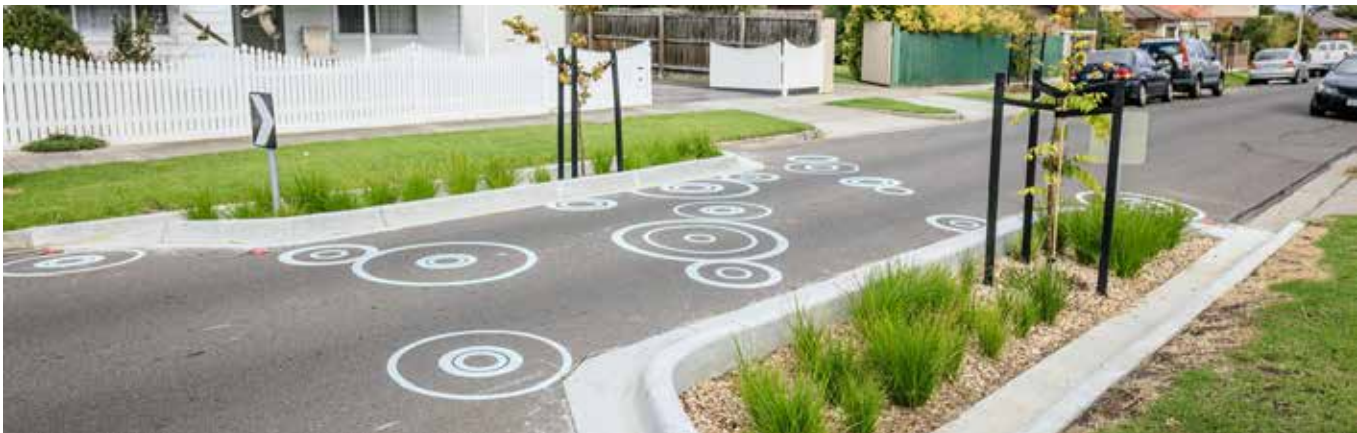
An example of lane narrowing in the City of Darebin (Image Credit City of Darebin).
