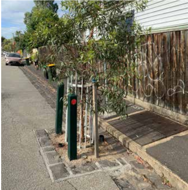
An example of a tree outstand with a flush bluestone kerb, rather than a raised kerb. Installed in Woodstock Street, Balaclava.
