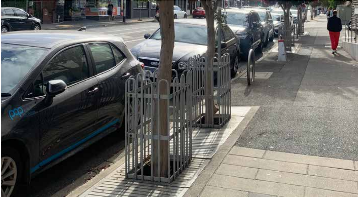
An example of tree cut outs on Carlisle Street with trees planted into pits large enough for connected soil between pairings.
