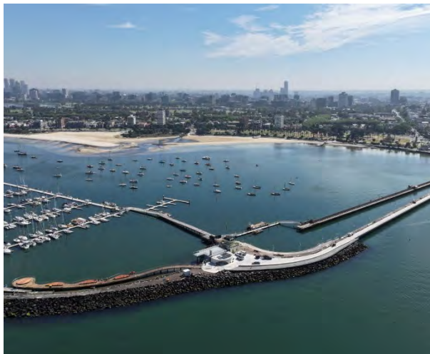
Upgraded St Kilda Pier (Source: Parks Victoria)
