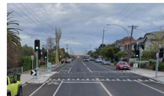
Raised Pedestrian Operated Signals
