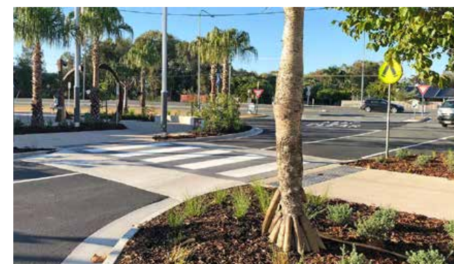
Tree planting in kerb extension improves streetscape greenery and pedestrian safety
