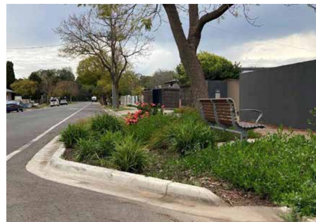
Rain garden within kerb extension filters runoff while providing green space and seating
