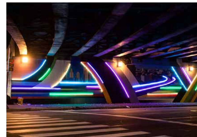
Underpass lighting brings colour and vibrancy to the streetscape
