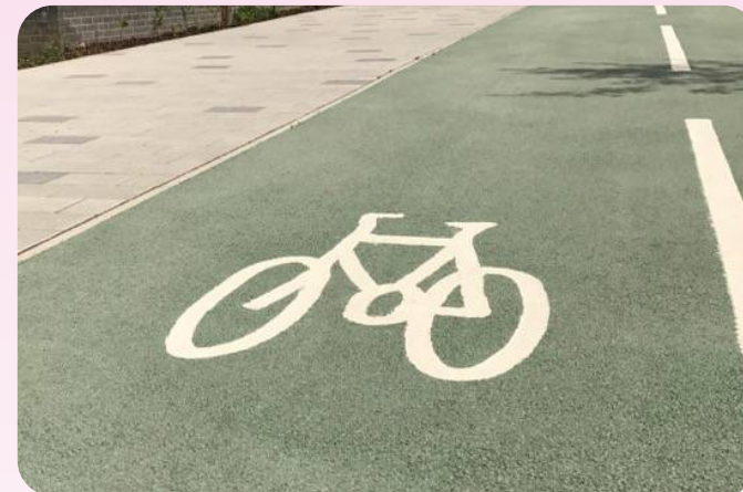
Dedicated bicycle lane with contrasting colour or surface material to visibly enhance cyclist safety
