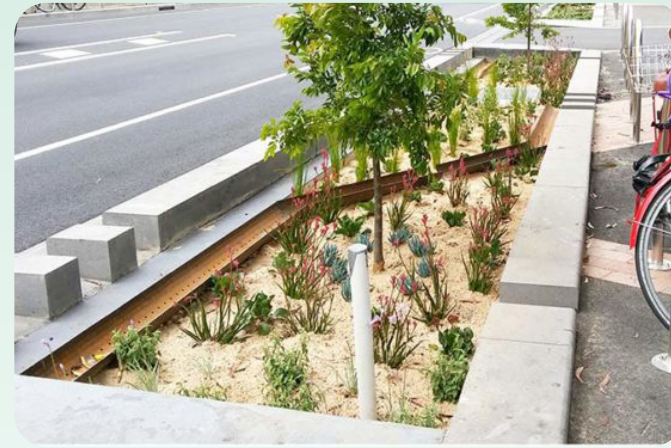
Rain gardens integrated into streetscapes for stormwater management and greenery
