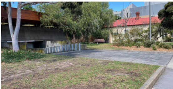
6 Lack of lighting in open spaces, such as behind the St Kilda Library, affects safety and visibility.
