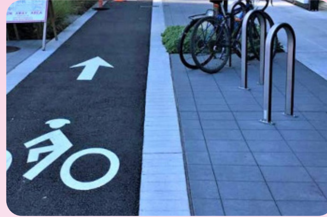
Bicycle parking provided level with bicycle path for ease of accessibility
