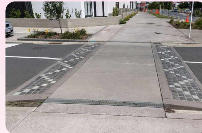
Raised pedestrian crossings for traffic calming
