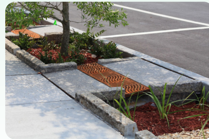
Biofiltration tree pits to reduce flood risks and improve tree health
