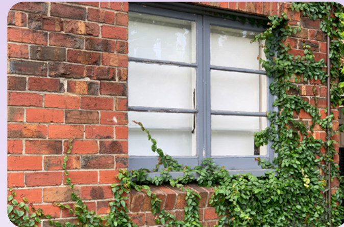
Green façades to soften built form and enhance the public realm
