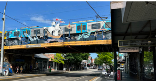
3 Many under-awning lights are not on or functioning reducing visibility along the footpath.
