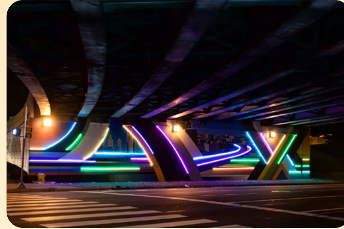
Underpass lighting brings colour and vibrancy to the streetscape.
