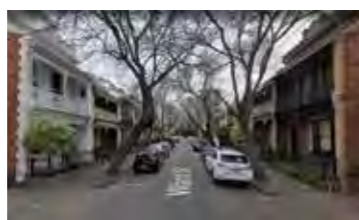
25 Dwellings per Hectare include terrace housing built up to the title boundary with little backyards and shared party walls.
