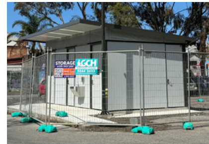
Newly constructed public toilet within off-street carpark
