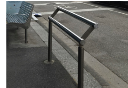
Existing pedestrian lean rail
