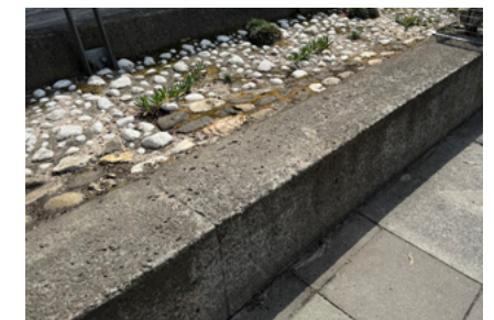
Existing concrete seat wall in front of the library
