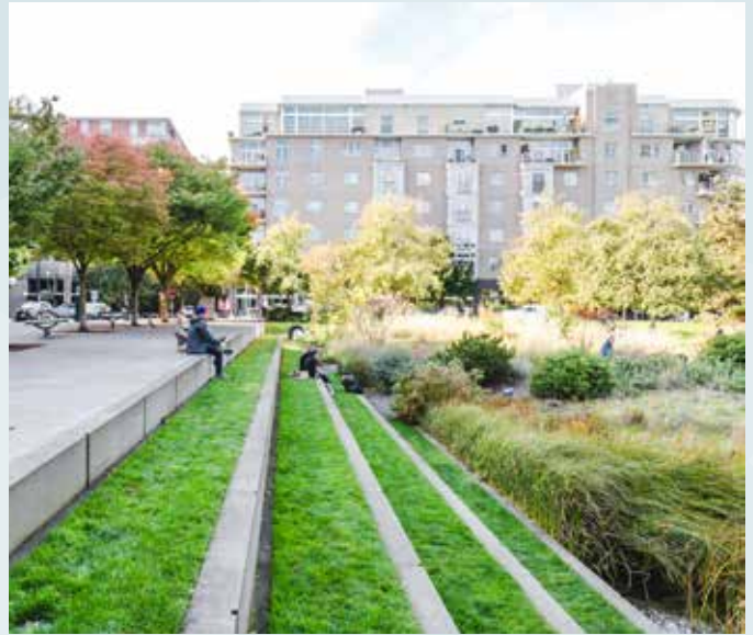
Designing public spaces to reduce the impacts of flooding - parks, sports fields and roads that retain water during severe storms.
