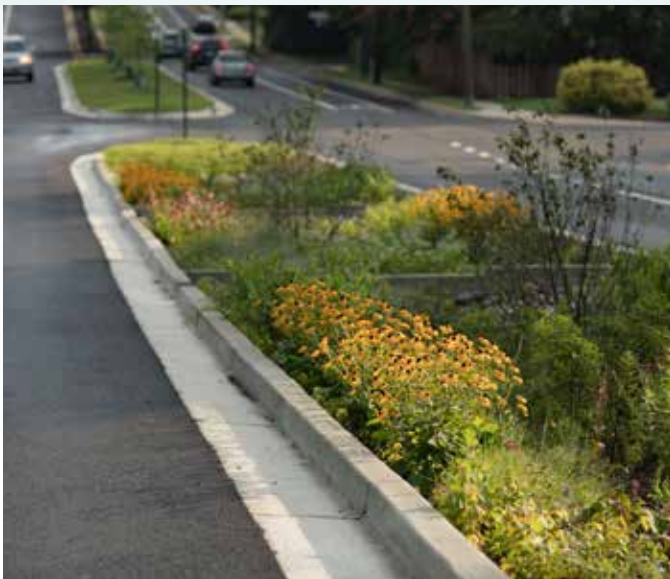
Raingardens capture and clean stormwater, are self-watering and enhance the amenity of our street spaces.
